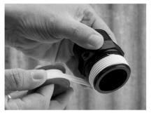
I. Apply PTFE tape or approved sealant to the male thread the blue handled ball valve is to be screwed in too.
